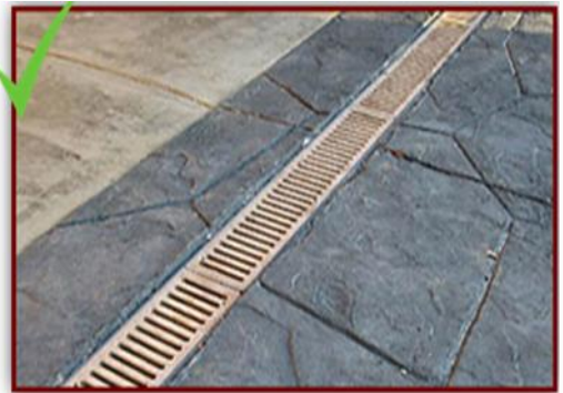
Fig 2.18 Floor with proper drainage
