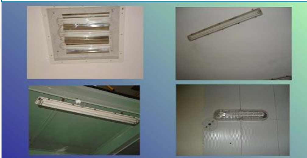
Fig 2.34. All lights in the process and packaging halls should be covered with shatter proof material to prevent any accidental contamination of product from shattered glass of lights
