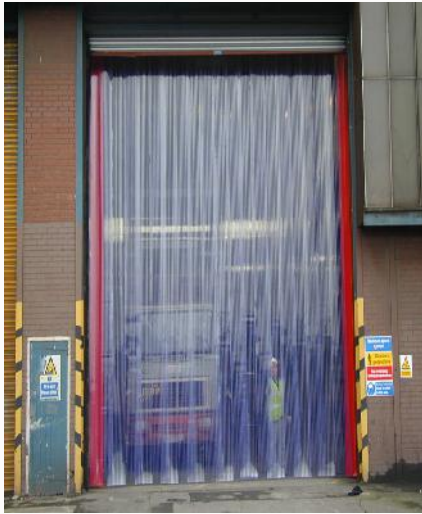
Fig 2.11 PVC Strip curtains
