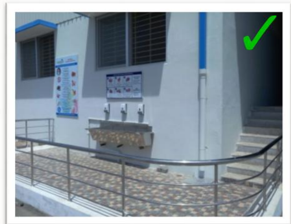
Fig.2.3 Plant entrance with hygiene station
