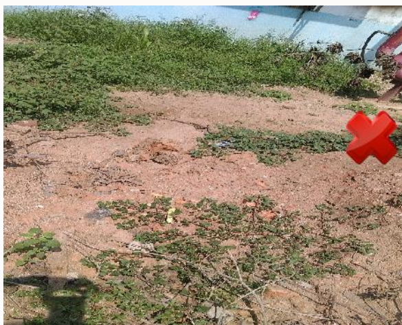
Fig.2.5 Vegetation growth near premises
