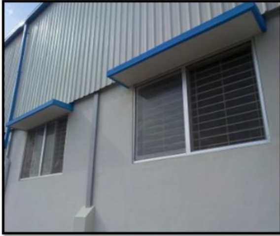
Fig.2.19 Netlons and mesh in window to avoid pest entry
